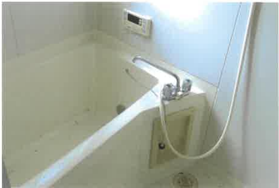
物件2:1階A号室浴室状況
