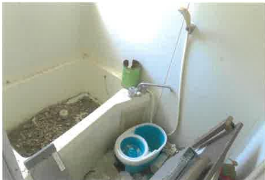
物件2:2階F号室浴室の状況
