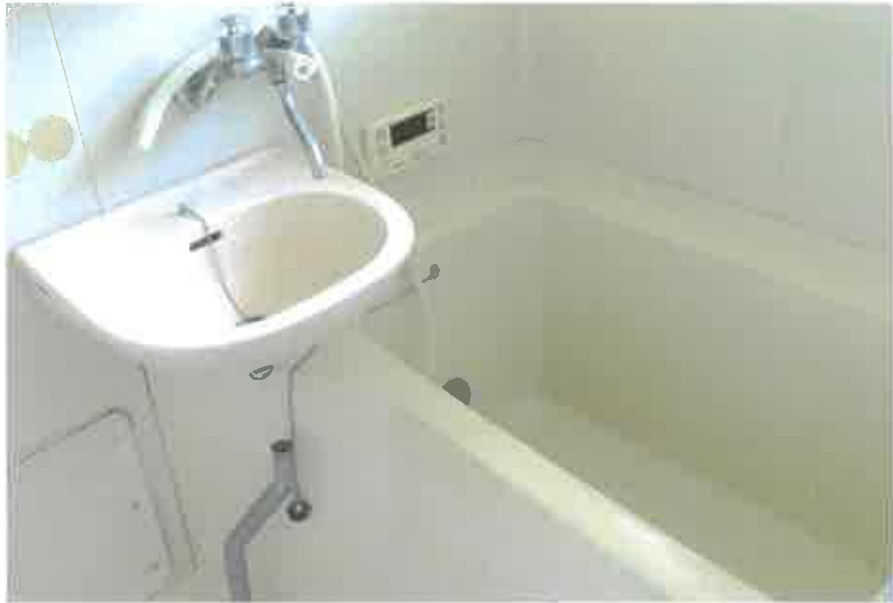
物件2:2階1号室浴室の状況
