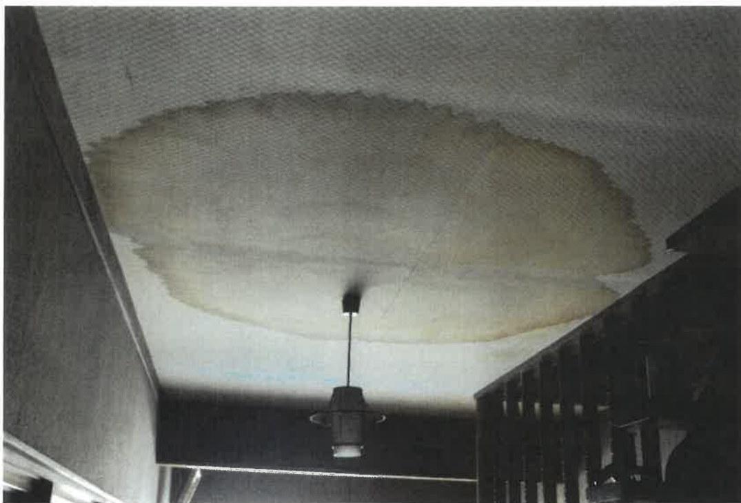
写真⑪ (物件2の玄関付近1階天井)
